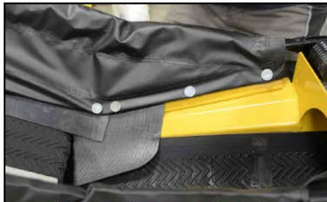
Fig 11 - Transition corner flashing in place
