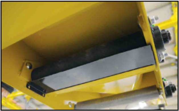
Fig 4 - Containment plate in place
