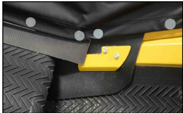
Fig 14 - Fasten flashing clamp
